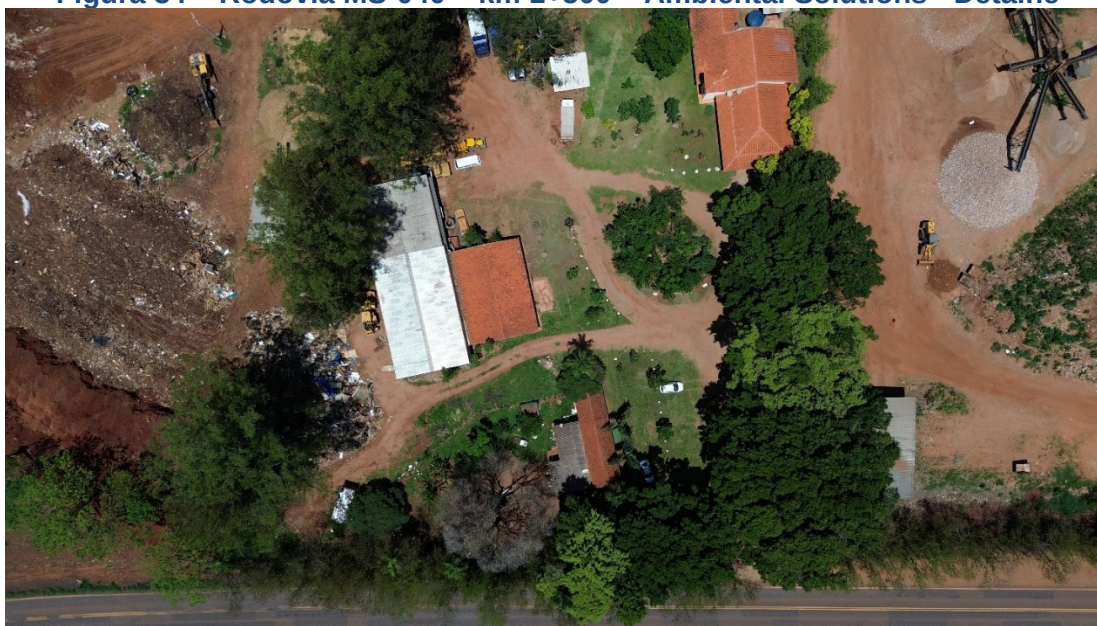
Figura 34 – Rodovia MS-040 – km 1+500 – Ambiental Solutions - Detalhe
