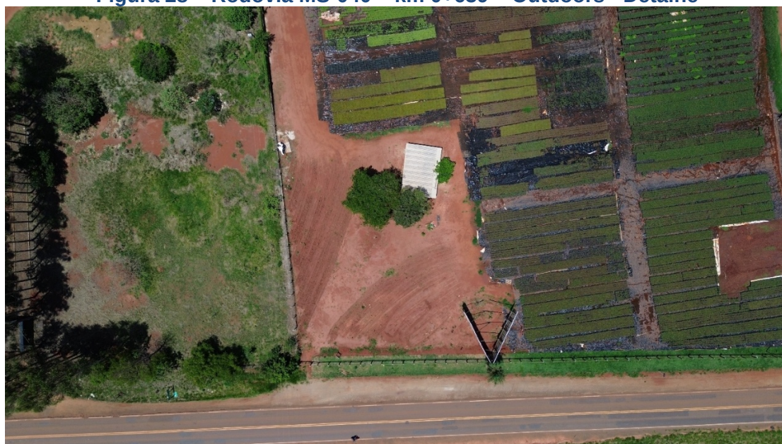
Figura 28 – Rodovia MS-040 – km 0+639 – Outdoors - Detalhe
