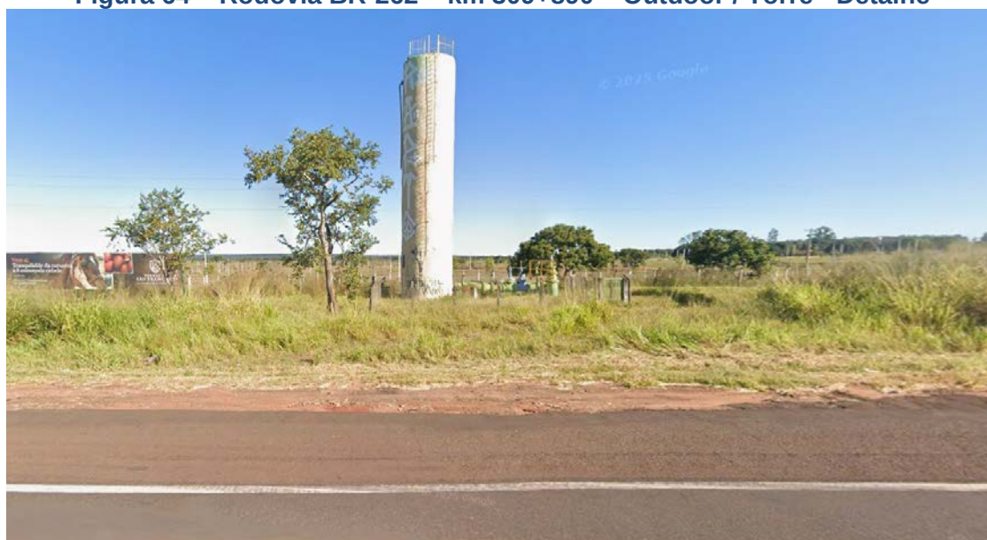
Figura 64 – Rodovia BR-262 – km 309+890 – Outdoor / Torre - Detalhe
