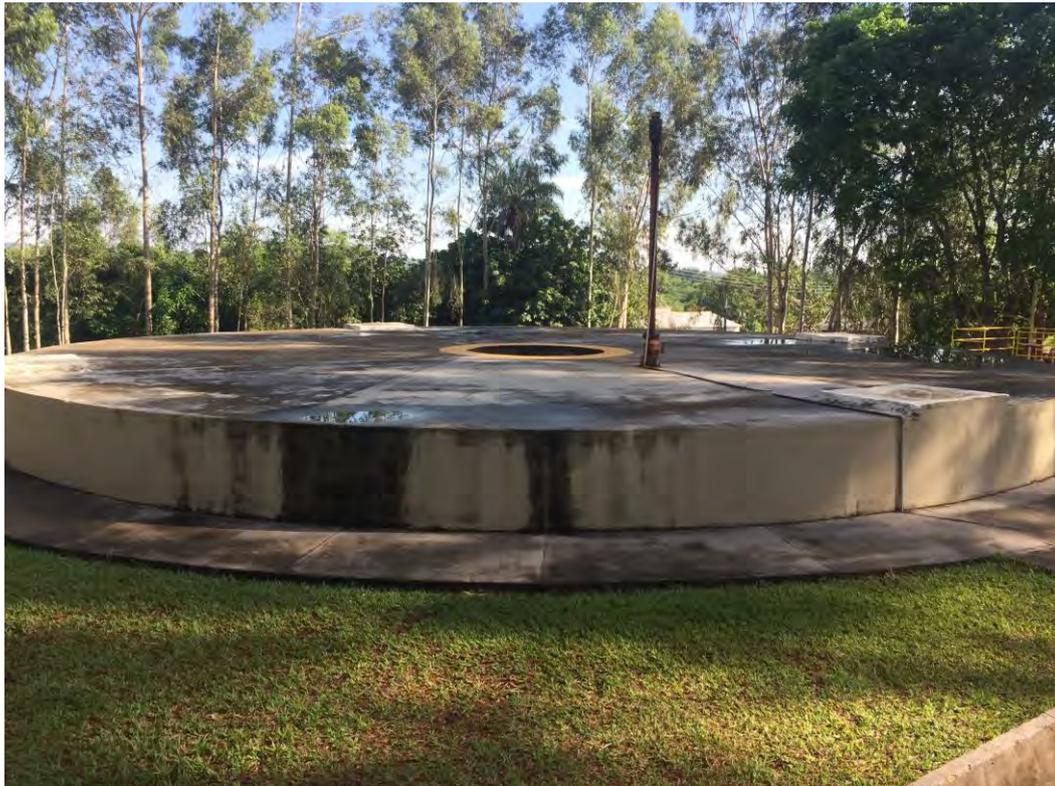
**Figura 15: Reator Anaeróbio (UASB).**
