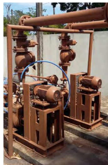
Conjunto de Recalque (Bombas Re-Autoescorvantes)
