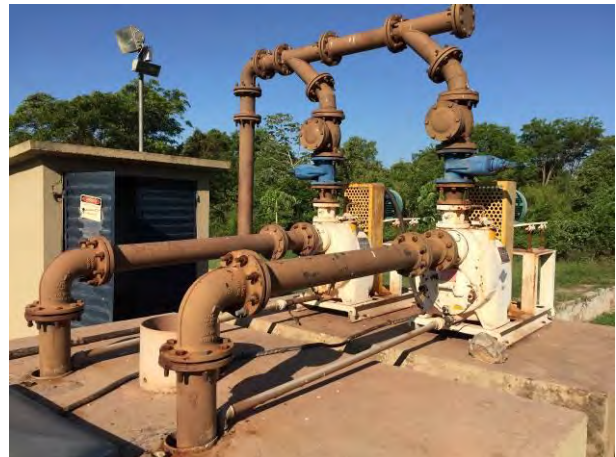
Barrilete de recalque
