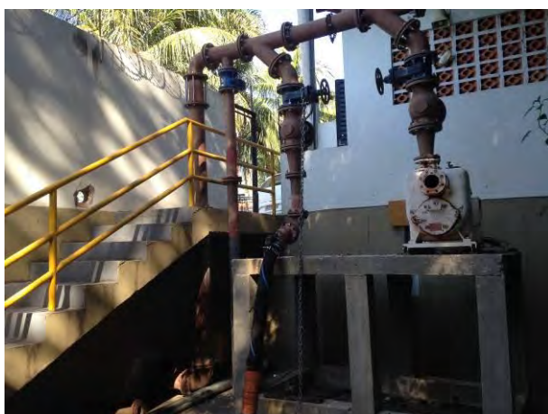
Barrilete de recalque
