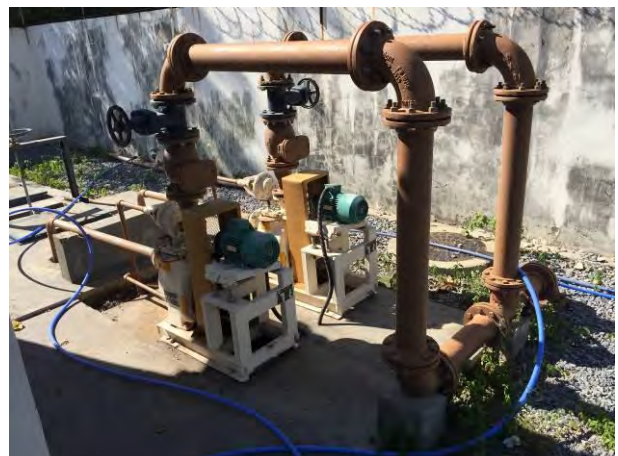
Barrilete de recalque
