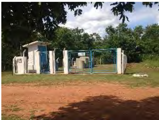
Fachada EEEB – 004 Guarapari
