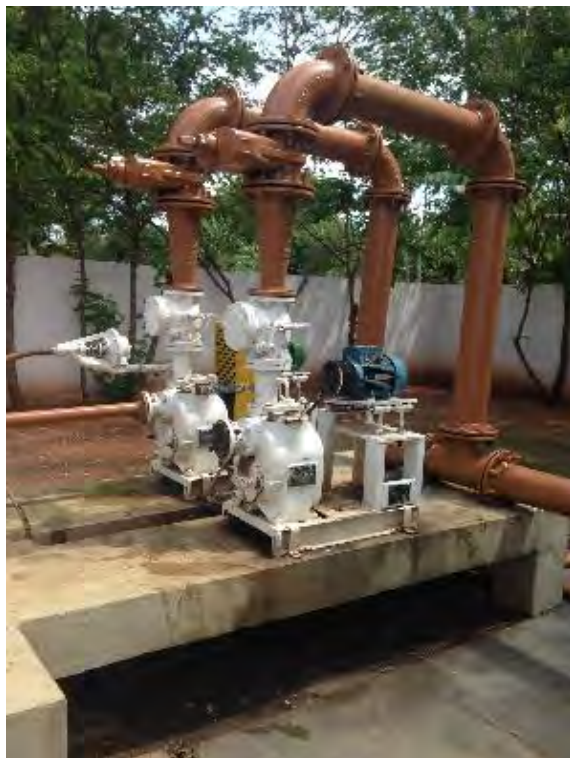
Bombas Re-autoeskorvantes e barrilete
