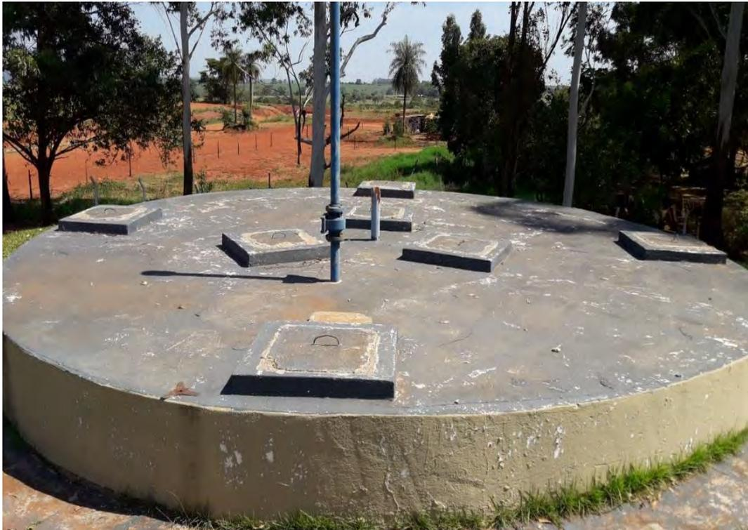
**Figura 23: Reator UASB.**
