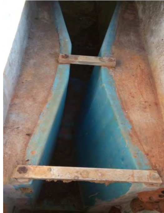
Calha Parshall, W= 3
