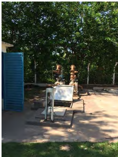
EEEB – Vista Frontal
