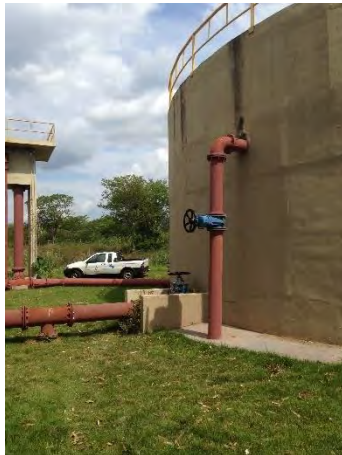
By Pass e Descarga de Lodo
